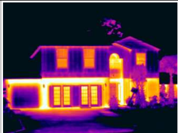
Description: IR Image #4 Thermal image of neighboring home with CBS construction showing considerably more heat loss
