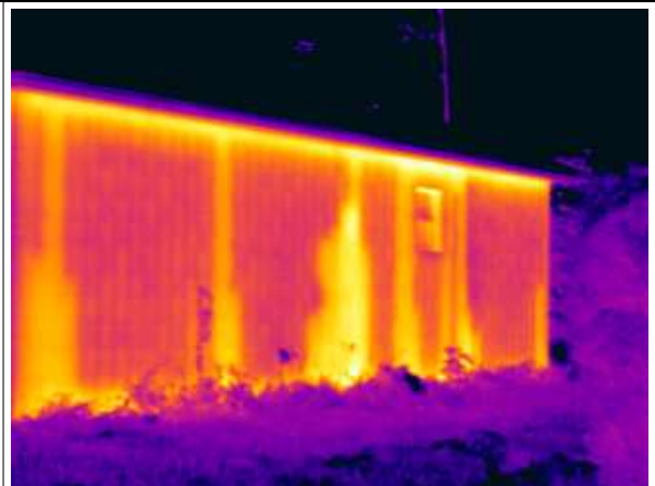
Description: IR Image #12 Thermal image of neighboring home with CBS construction showing considerably more heat loss
