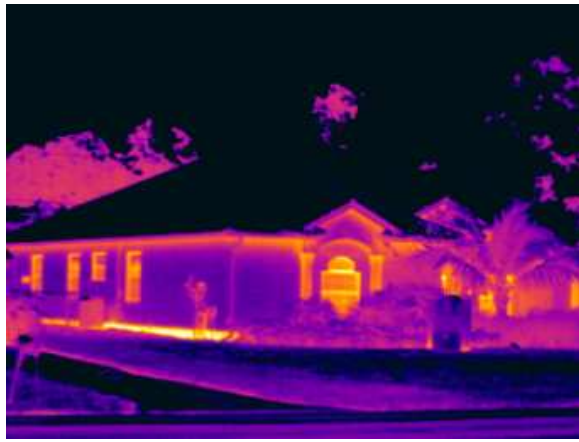
Description: IR Image #1 Thermal image of ICF construction
