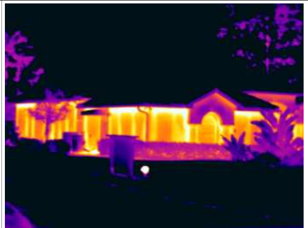
Description: IR Image #16 Thermal image of neighboring home with CBS construction showing considerably more heat loss
